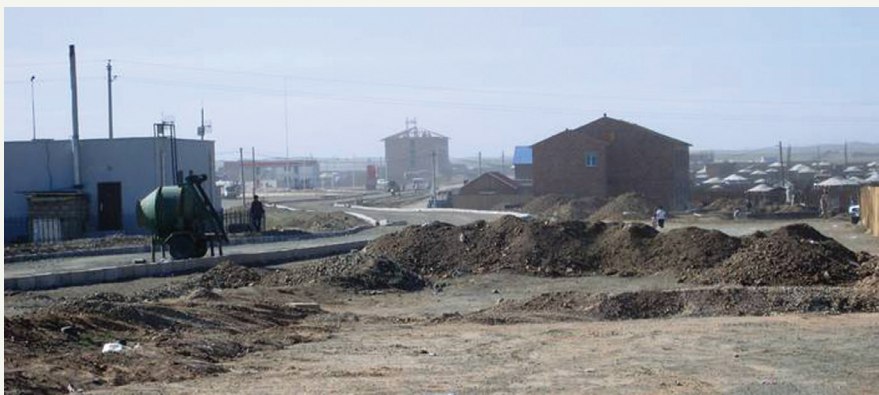
Tsogtsetsii Soum, road construction 2011
