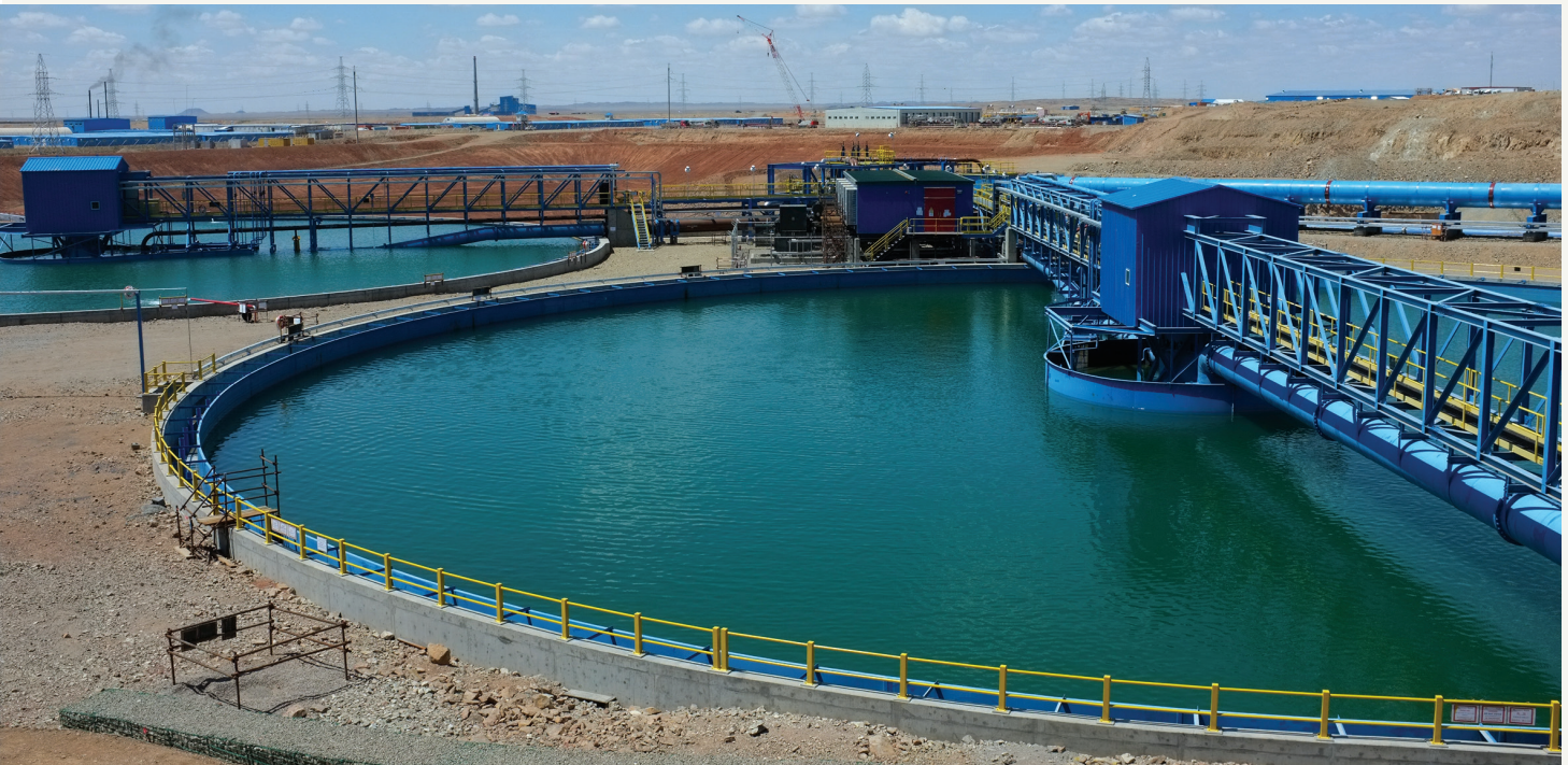
Oyu Tolgoi, water treatment facility (Photo Source: GIZ's IMRI)
