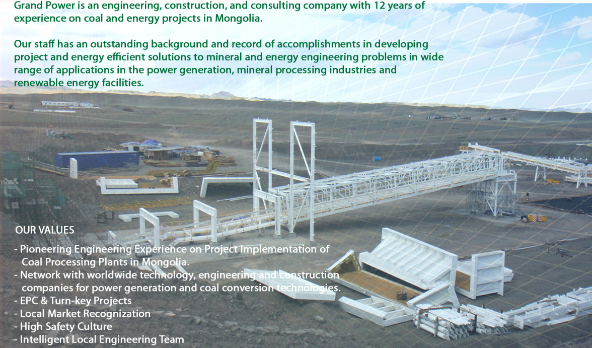
COAL HANDLING AND DRY PROCESSING PLANT
