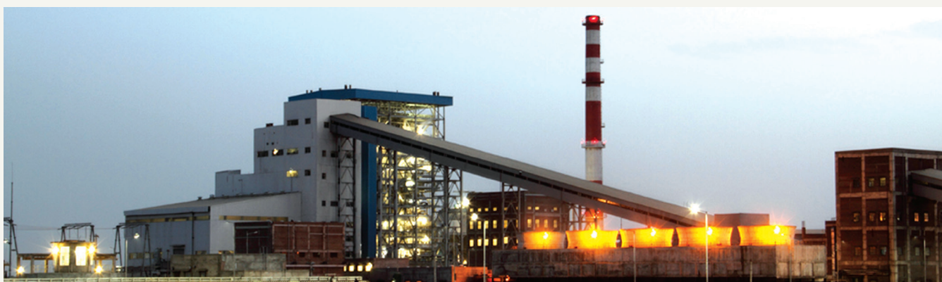
Tavan Tolgoi Power Plant
