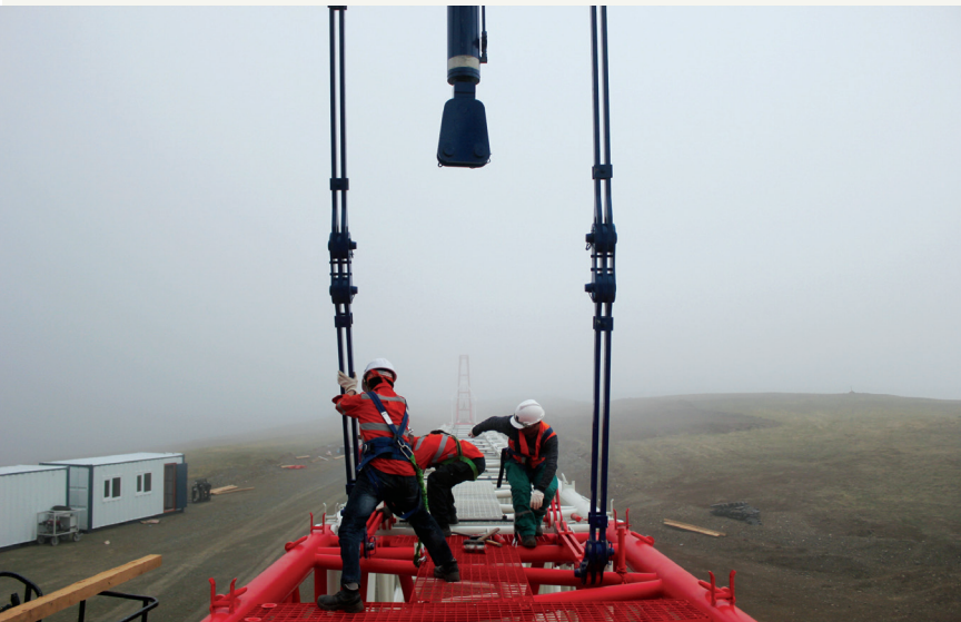
A 650 tonne mobile crane
