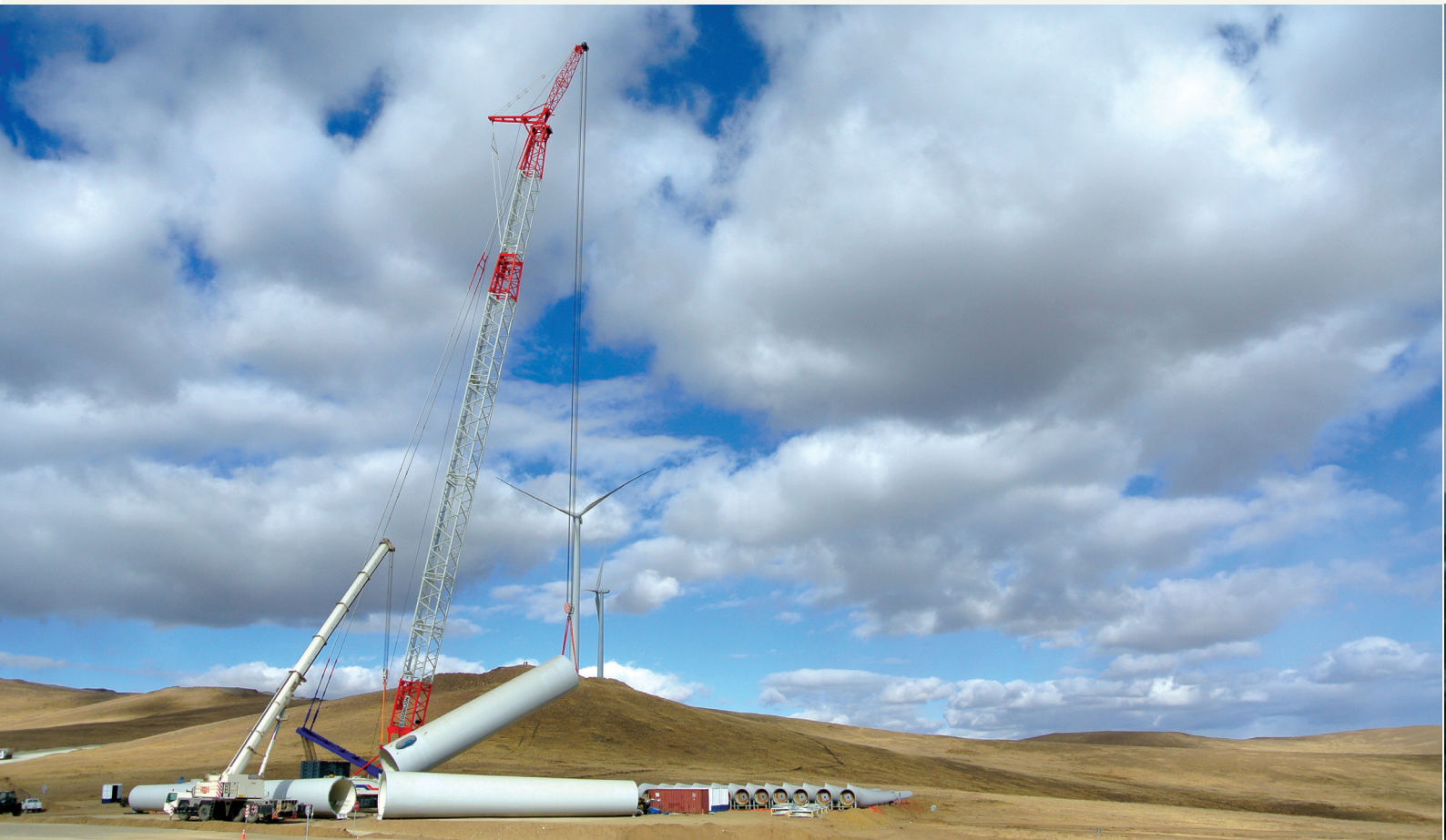
Installation of tower
