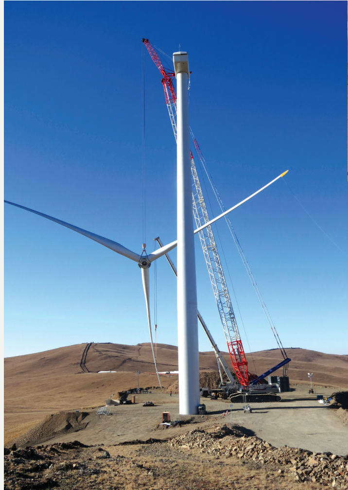
Installation of blade
