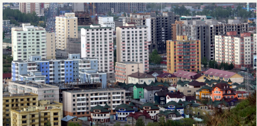
Construction industry has 125 percent growth compared to the previous year
