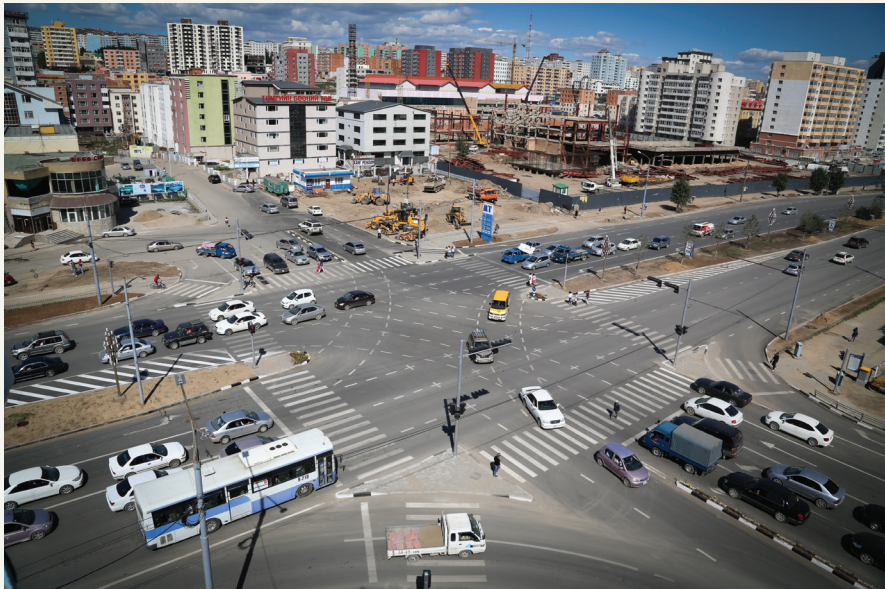
A new four-way intersection as a part of Gudajm (Street) project
