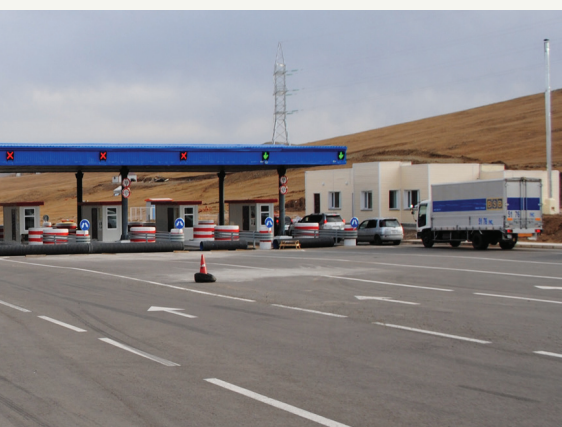
Renovation of the traffic checkpoint in the west of Ulaanbaatar
