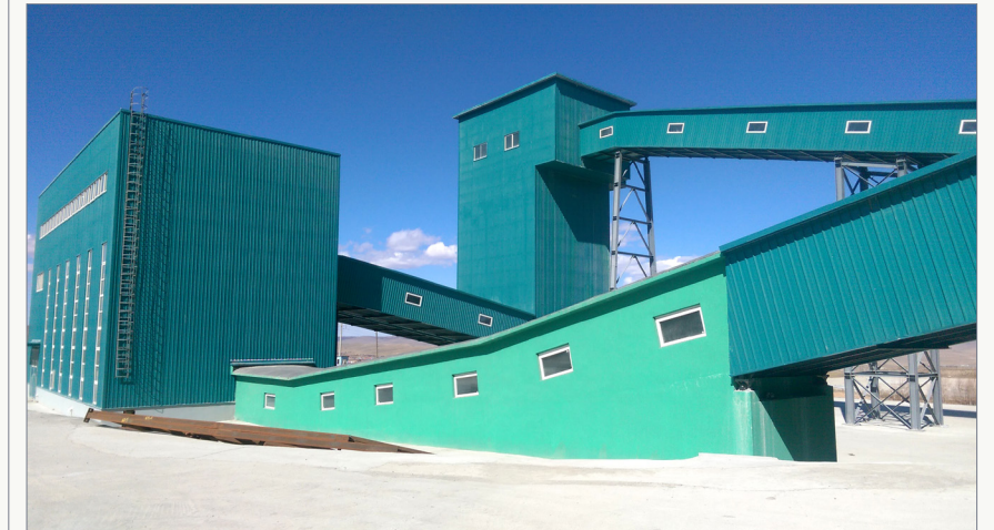
The expansion of the autogenic grinding circuit
