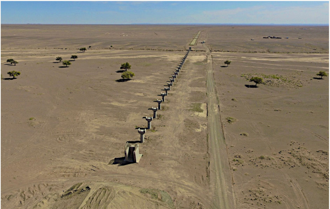
The Ukhaakhudag-Gashuunsukhait railway will comprise 15 bridges, 14 tunnels and two stations.
